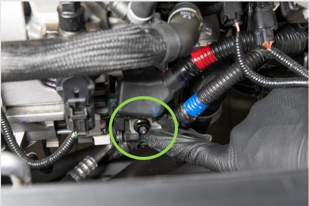
STEP 7 - Disconnect -48V terminal from the iBSG
