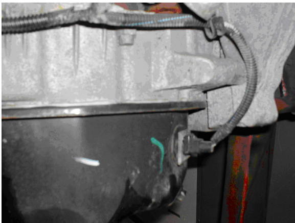
Figure 65 Low Oil Level Switch (Disc 1)
